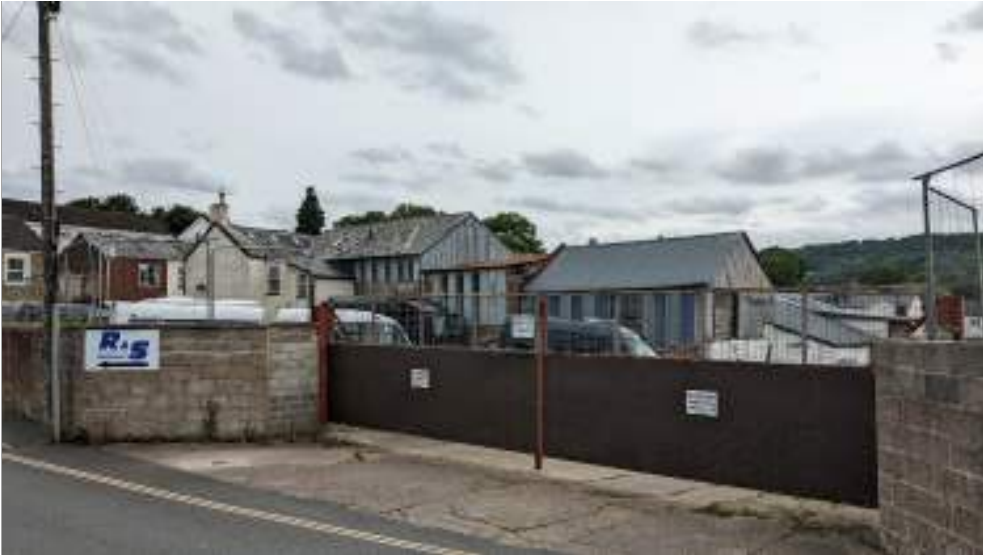
Site existing condition, view from King Street
