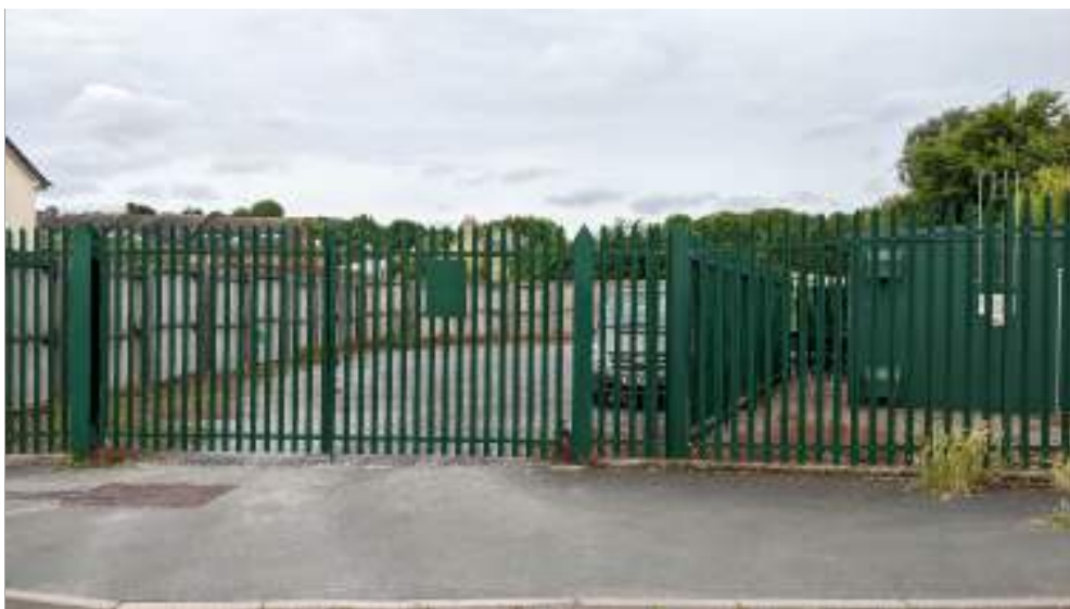
Site existing condition, view from King Street
